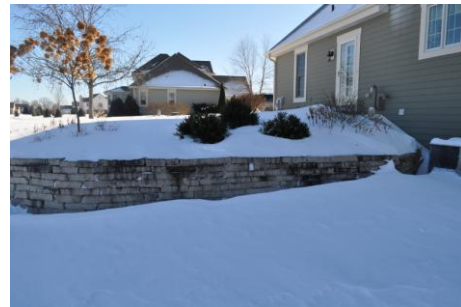
The retaining wall is in good shape. The moss and mildew gives it character.
