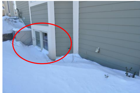
Remove the snow from the window sill. This will stop the acceleration of wood rot.
